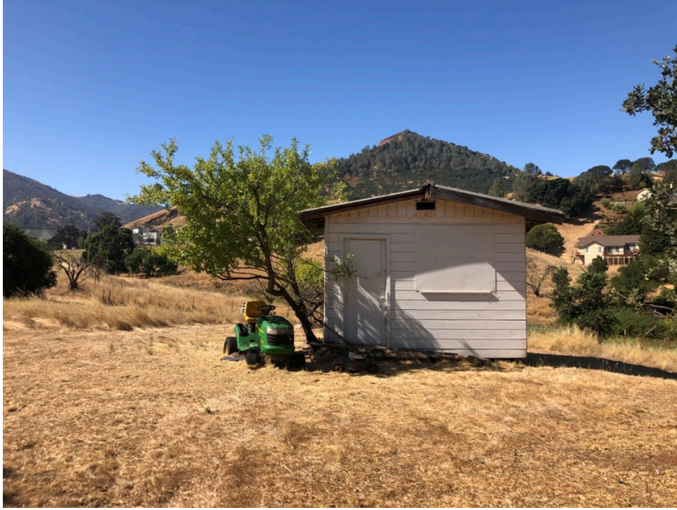
7. View of shed on northwest portion of subject property
