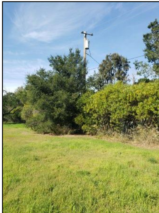
6 : View from northern parcel looking towards the northwest. Background depicts electrical transformer along the northern property boundary.
