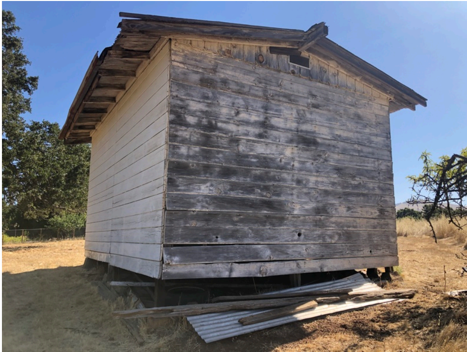
8. View of shed on northwest portion of subject property
